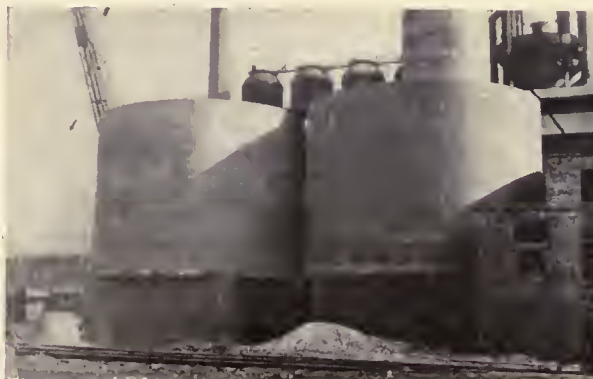
WATER PURIFYING TANKS
